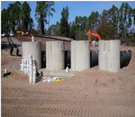
Risers, 48-in Drainage Pipes
