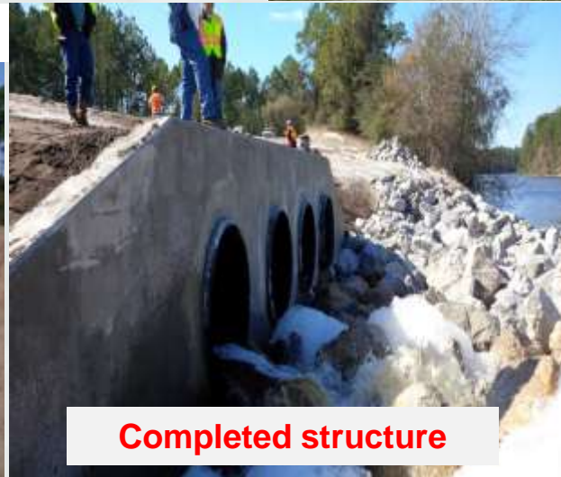
Risers, 48-in Drainage Pipes
